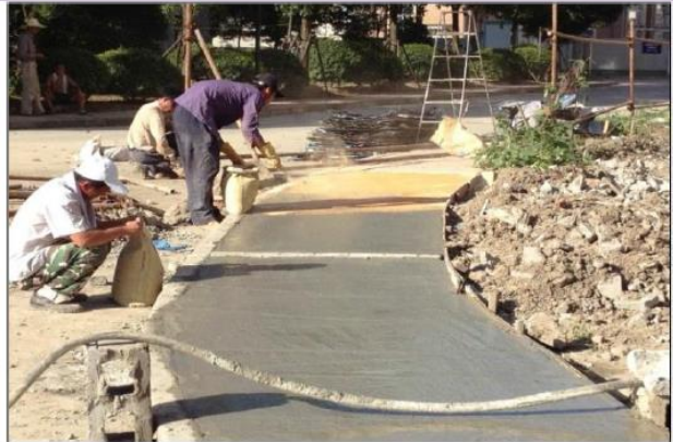
Step 2: Casting color hardener on the cement floor, normally 3-4kg on 1 square meter.
