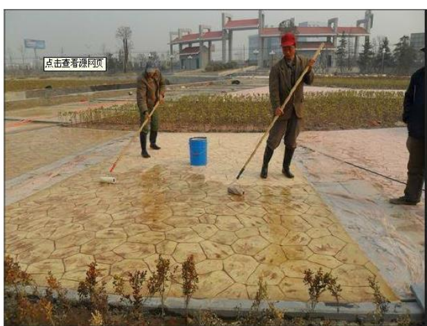
Step 6: Hold 3days for curing, then spray sealer on the floor, 0.2kg on 1 square meter.
