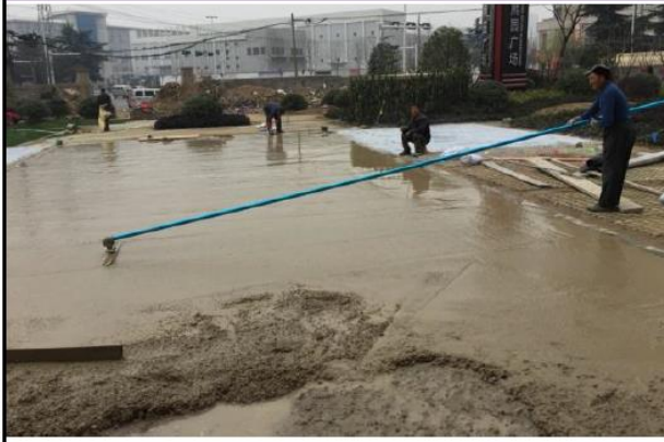
Step 1: Making the wet cement floor to even, no water hole on the surface.
