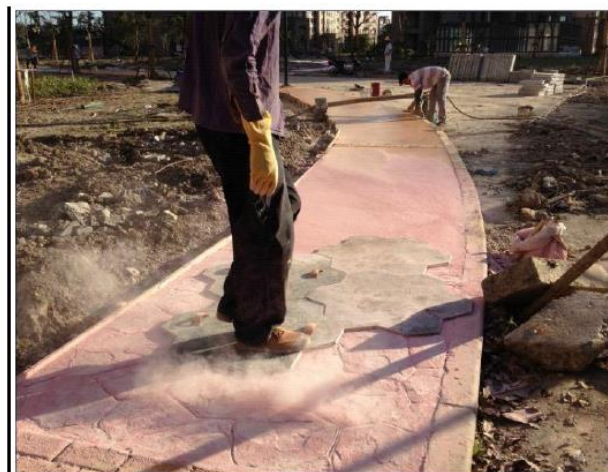
Step 5: Stamping the floor with concrete stamp mat and Plate Temper.
