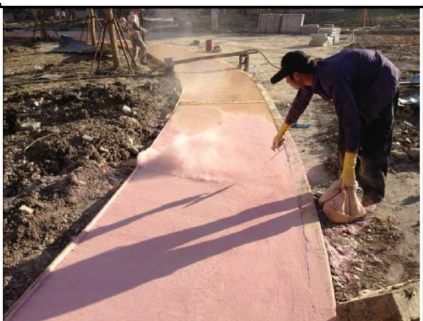
Step 4: Casting release agent on the floor, normally 0.15kg on 1 square meter.
