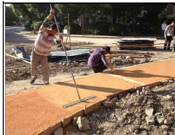
Step 3: when the color hardener is humid, making the floor smooth with bull float.
